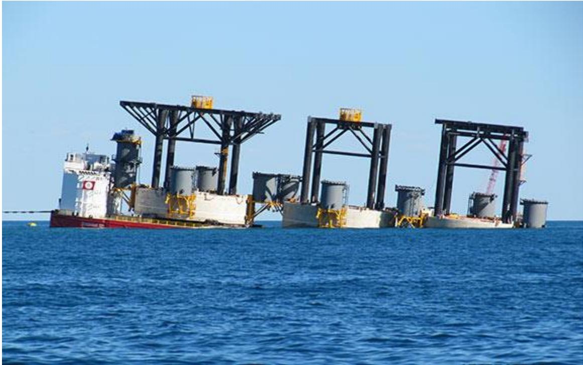
Caissons on a barge travelling to the design location.
